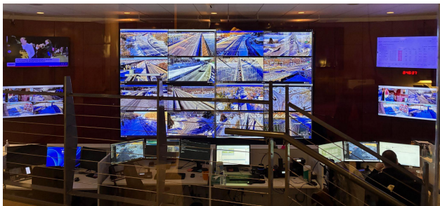
Figure 8 - NYSBA Command Center for 5 toll bridges over the Hudson River in New York State. Staffed 24/7. Vessel collision dashboard, marine radio, and traffic gate control are being deployed here.
