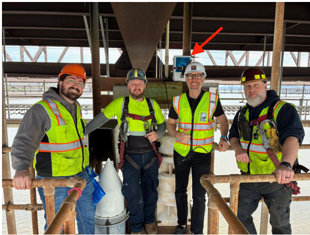
Figure 7 - Hardware Unit for Vessel Collision Warning System (See Arrow) at the Newburgh-Beacon Bridges over the Hudson River in New York State. NYSBA Project Manager, NYSBA Bridge Mechanics, and the Author smiling after completing the installation and successfully testing functionality.
